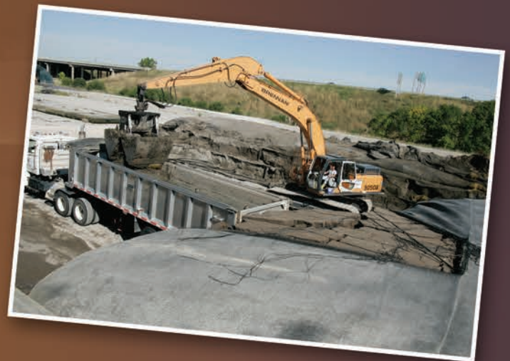
Dewatered sludge being removed from a Geotube® container with a backhoe
