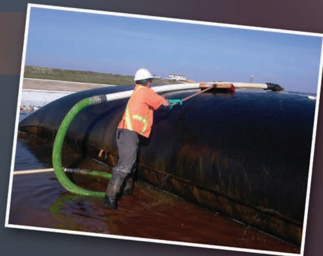
Our skilled installation crews provide fast and efficient installation services
