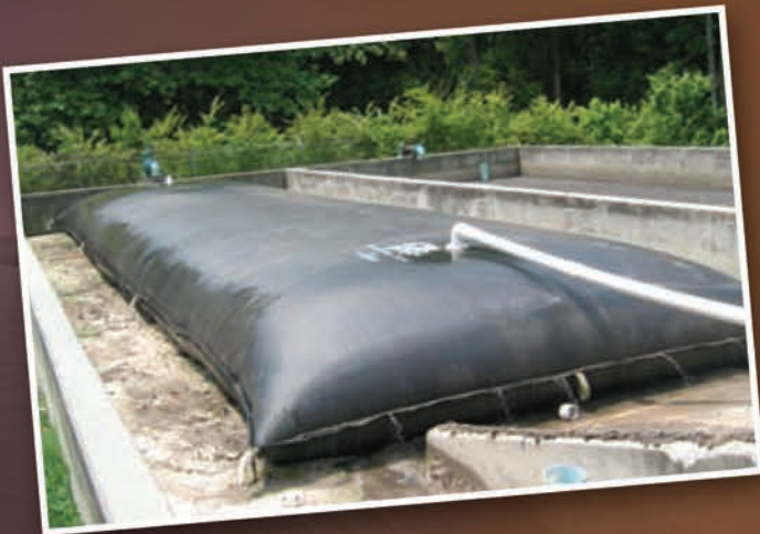
Geotube® unit in municipal wastewater treatment drying beds
