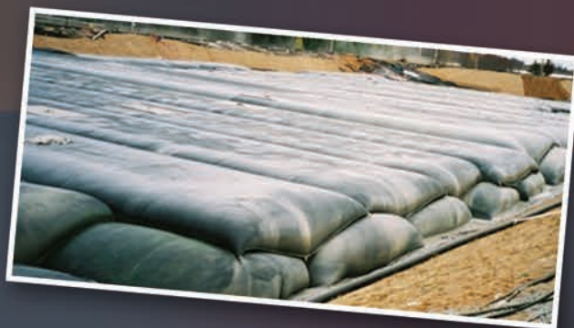
Geotube® containers in activated sludge basin at paper plant
