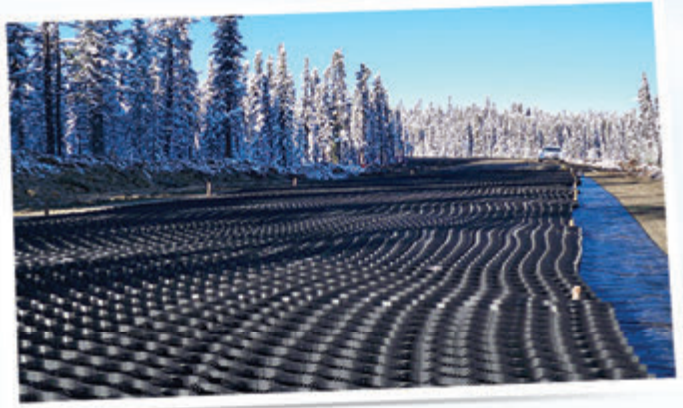
Site access road built over muskeg using the Geoweb® system
