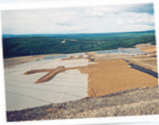
This heap leach pad liner used prefabricated geomembranes to meet development schedules in a remote location.
