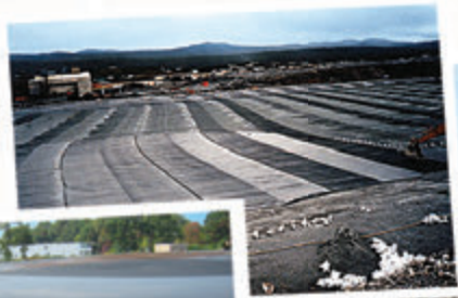
High strength geotextile pond closure for a white phosphorus sludge pond cover. The geotextile supported a permanent earthen cover.
