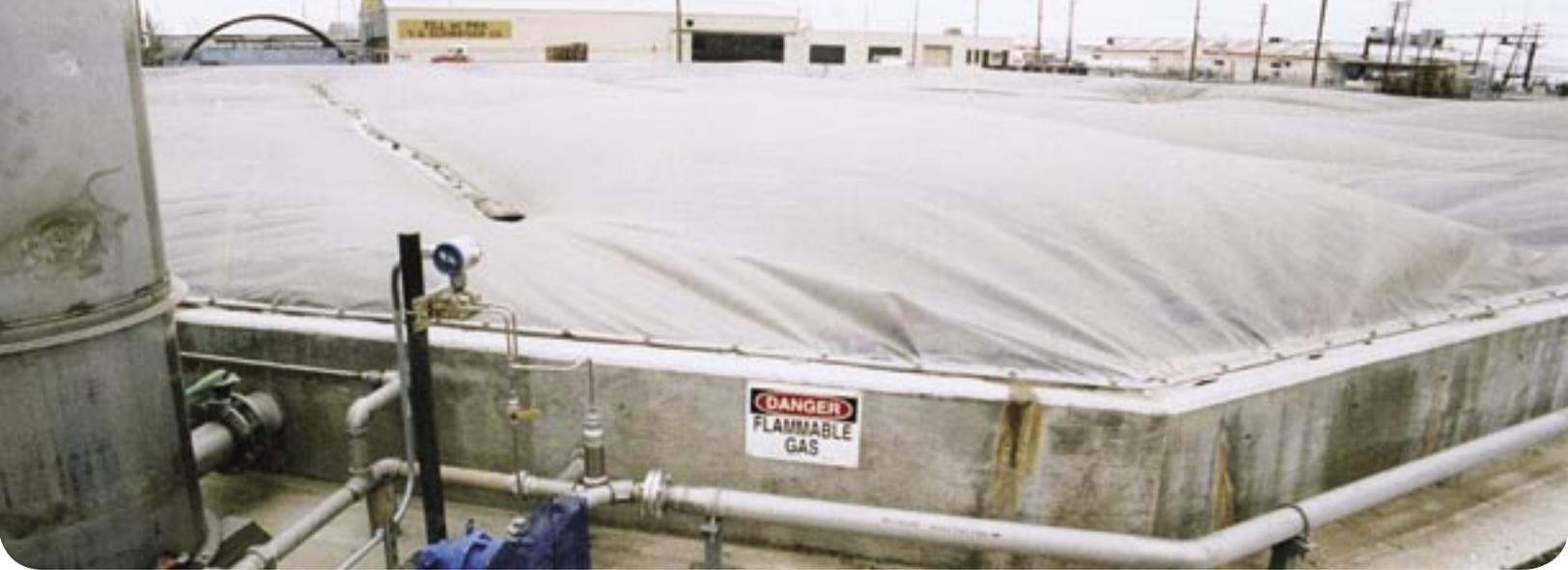
**Our prefabricated gas collection covers are made from a new fabric-supported polyolefin that has the strength and flexibility needed for gas collection.**
