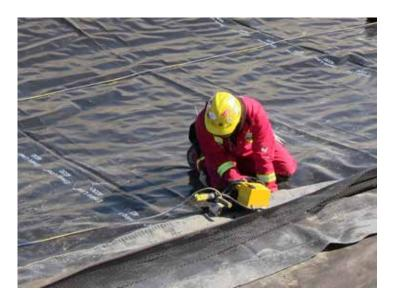
production welds. If they are performed as part of a detail or repair, they shall be recorded on the Geomembrane Detail & Test Log (Appendix E).
