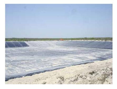
**9.3.2.** All details must be constructed using equipment that has been through the Qualification Weld process, and follow the applicable welding procedures.
