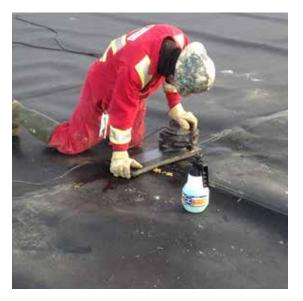
**8.2.3.3.1.** Ensure that this procedure does not puncture or otherwise damage the sheet material, seams or welds, but enough pressure is applied to perform the test.
