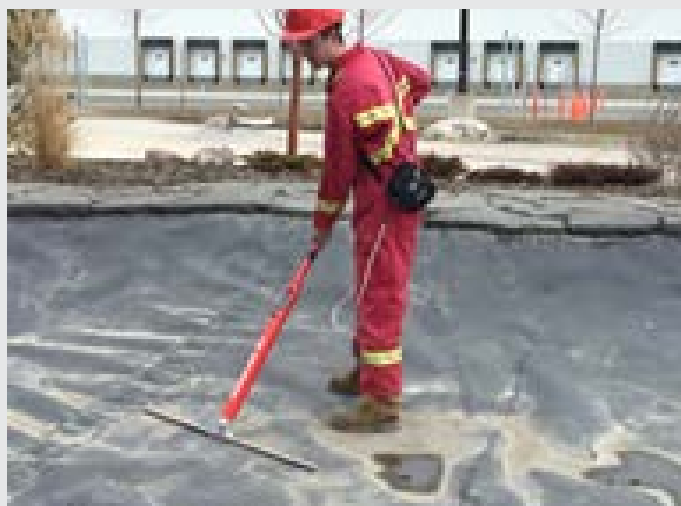
Figure 5. Arc Testing on an exposed geomembrane
