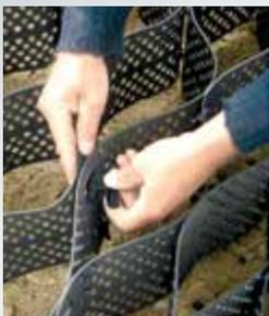
For quick and easy connection of GEOWEB® sections, exclusive ATRA® keys significantly reduce contractor installation time and provide a three-times-stronger connection of GEOWEB® sections.
