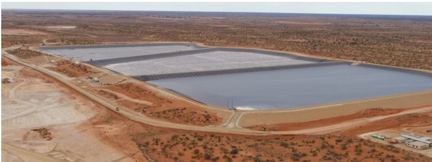
Figure 3. The completed storage facility in operation.
