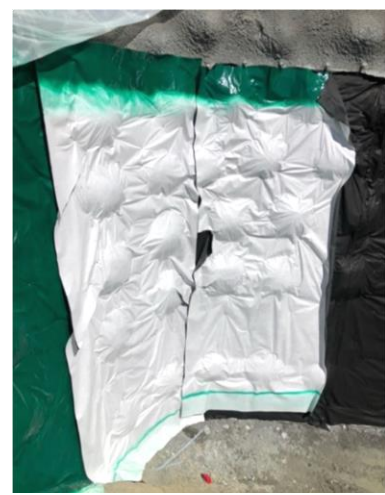
Figure 3. Conforming the Geotextile into A Corner
