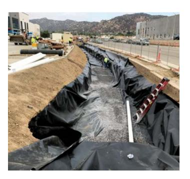
Also known as infiltration swales, Bioswales are a form of bioretention designed to slow surface water runoff and help remove stormwater pollutants. These low-maintenance systems transport large volumes of stormwater to a discharge point, slowing the velocity and filtering the water.
