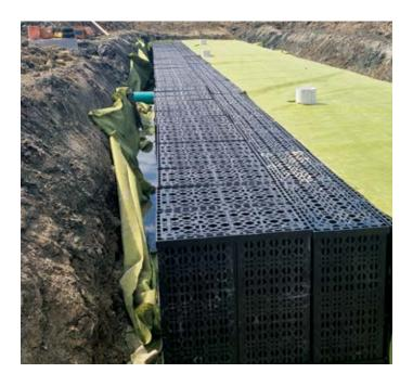
NuBarrier™ is an innovative nonwoven geotextile designed with the added benefit of microbial digestion of hydrocarbons. Its unique green color also acts as a warning barrier to protect your infiltration assets. The geotextile accumulates a biofilm that functions to biologically decontaminate hydrocarbons at a rate of up to 400 grams per m² per year, ideal for use under parking lots and within bioswales.
