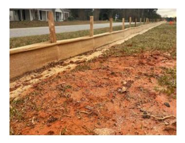
Quickly and cost-effectively contain and treat sedimentladen flow with the newest innovative solution developed by Western Green. Combining the best features of wattles and silt fences, WattleFence™ replaces traditional technologies for perimeter control, slope interruption, ditch checks, and more.
