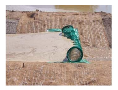
Prevent sediment-laden water from entering storm systems with a Layfield spring berm. When used in channels and highway ditches these sediment control devices reduce the flow velocity of water and help to reduce erosion by filtering out and trapping silt and sediment.
