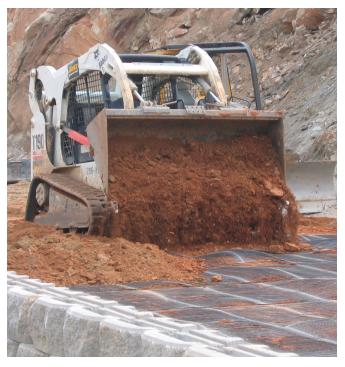
Tensar UX Geogrids install easily in stand alone applications as well as in conjunction with one of our proprietary soil stabilization systems.
