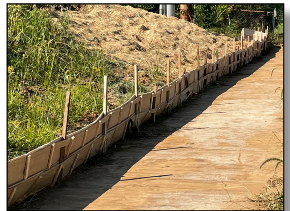
Shown Above: WattleFence under channel flow, schematic of WattleFence, Double layer of WattleFence installed as a stockpile perimeter control.
