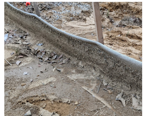
Shown Left to Right: WattleFence as a sediment barrier along a riverbank, WattleFence in action under sediment-laden flows, WattleFence continued performance after multiple flow event.
