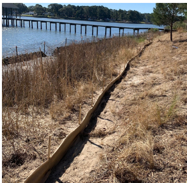
Shown Left to Right: WattleFence as a sediment barrier along a riverbank, WattleFence in action under sediment-laden flows, WattleFence continued performance after multiple flow event.
