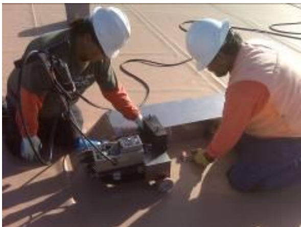
Figure 5: Fabrication of Sump Floats
