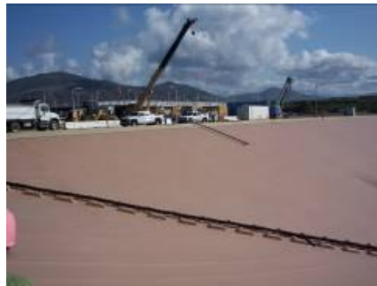
Figure 4: Installation of Pipe System
