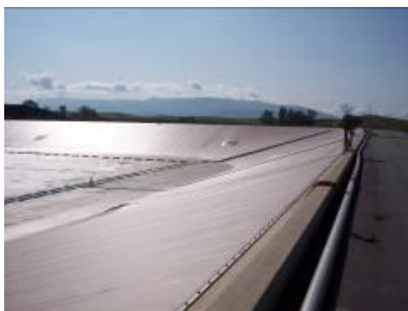
Figure 6: Mechanical Anchorage Detail
