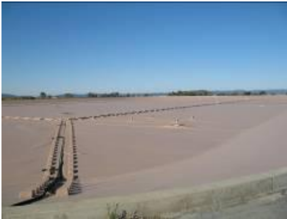
Figure 1: Overview of Floating Cover
