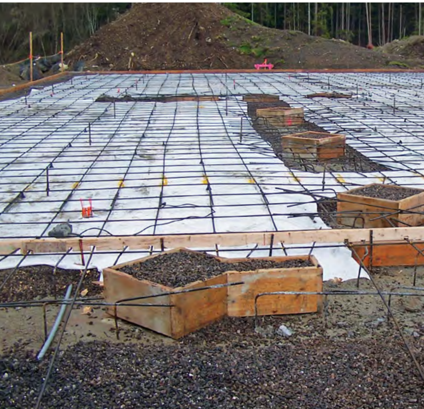
Figure 7: Cut a patch large enough to overlap 12" in all directions and slide over penetrations. (Make openings as tight as possible.)
