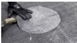
Figure 2: Heat-tack Geovolt® Nonwoven.
