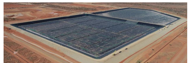
Figure 7. Photo of installed bi-modal HDPE in BHP EP7
