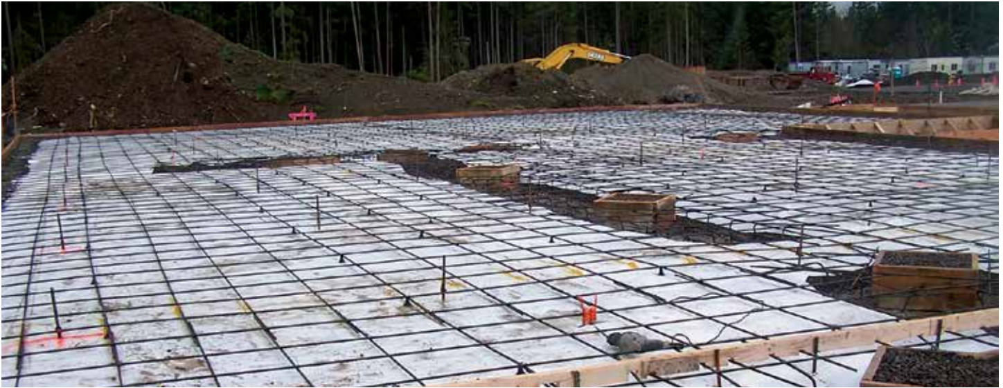
Figure 14. VaporFlex™ Standard underbuilding application.
