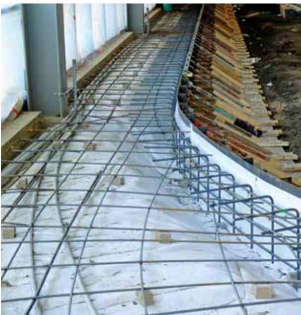
Figure 1. VaporFlex® Standard installation
